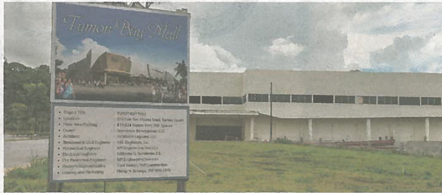
The Tumon Bay Mall building stands silent in Tumon on Thursday. RICK CRUZ/PDN
